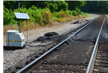
Flange grease is applied to the gauge face of the rail before entering curve
