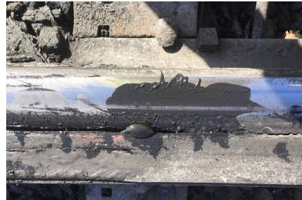
TOR Friction Modifier is applied on top of rail
